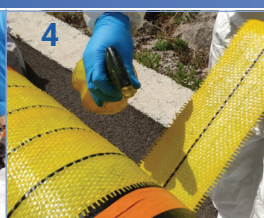
R1D wrapping (spray water continuously)
