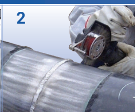
Surface preparation Sa2½ / St3 & roughness Rz > 60 µm (2.4 mil)
