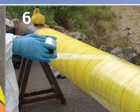
Compression film application and perforation
