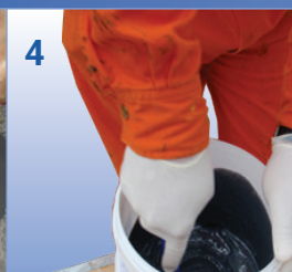
4 3X bi-component epoxy resin preparation
