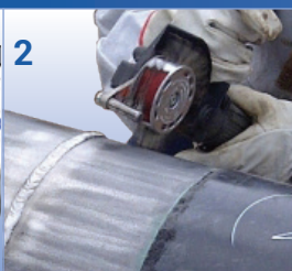
2 Surface preparation Sa2½ / St3 & roughness Rz > 60 µm (2.4 mil)
