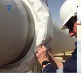
Leak sealing with soft cover application and valve
