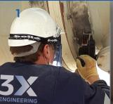
Surface preparation Sa2½ / St3 & roughness Rz > 60 µm (2.4 mil)
