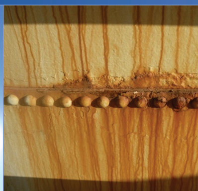
INTERNAL CORROSION
