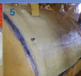
5 Kevlar® patching with 3X resin application
