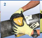
Install the STOPKiT® and slide it over the leak
